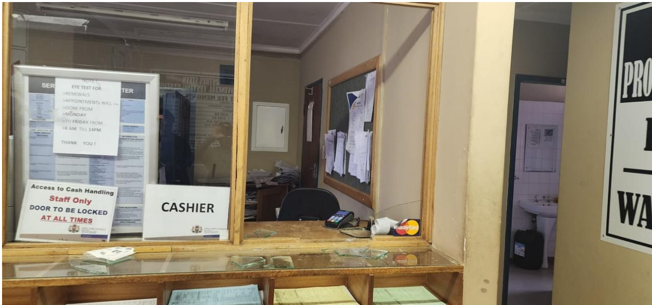
Figure 5. Heilbron Licensing centre vandalised & computers stolen - Photo supplied by HOD Tshabalala
